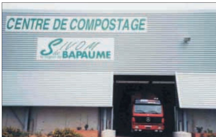
Above: Central composting facility
